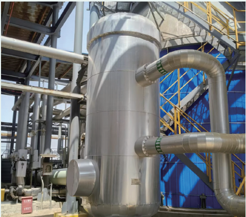
Figure 5-8 Desulfurization slurry waste heat recovery project in thermal workshop
