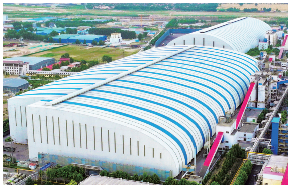
Figure 5-10 Fully Enclosed Coal Yard
